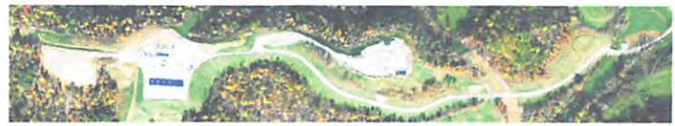
Site is fully stabilized.
