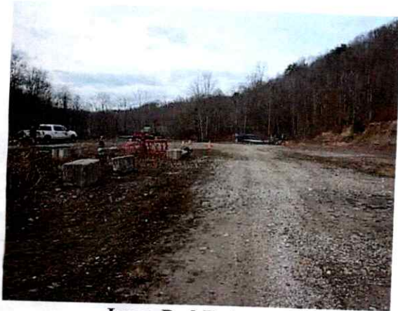
Jones Pad Entrance
