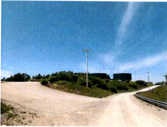
Berger A 3H Well Pad Site
