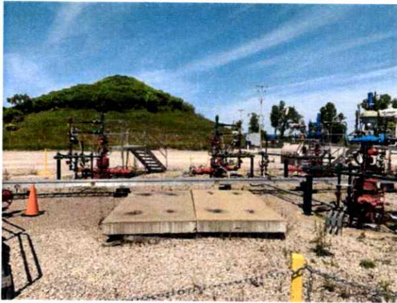
Berger A 3H Well Pad Site
