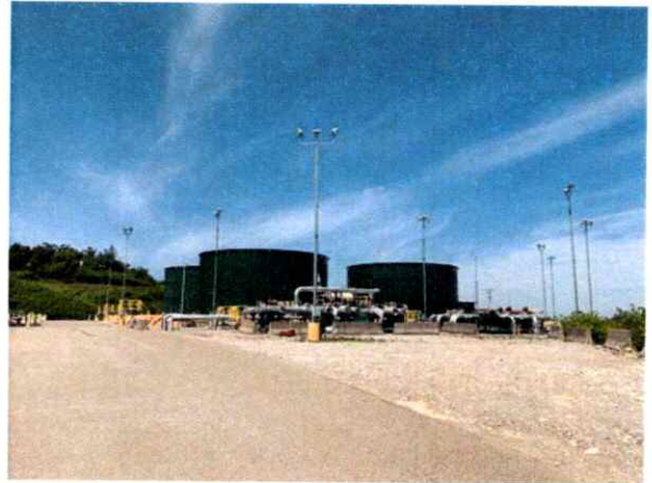
Berger A 3H Well Pad Site
