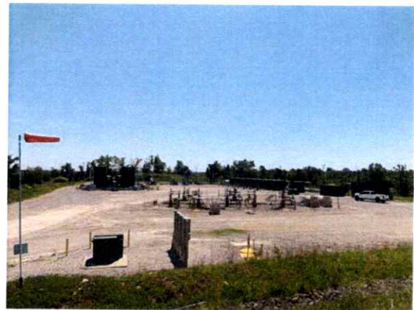
Berger A 3H Well Pad Site
