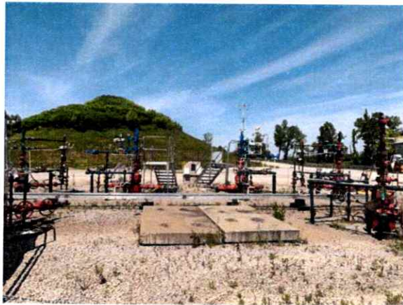
Berger A 3H Well Pad Site
