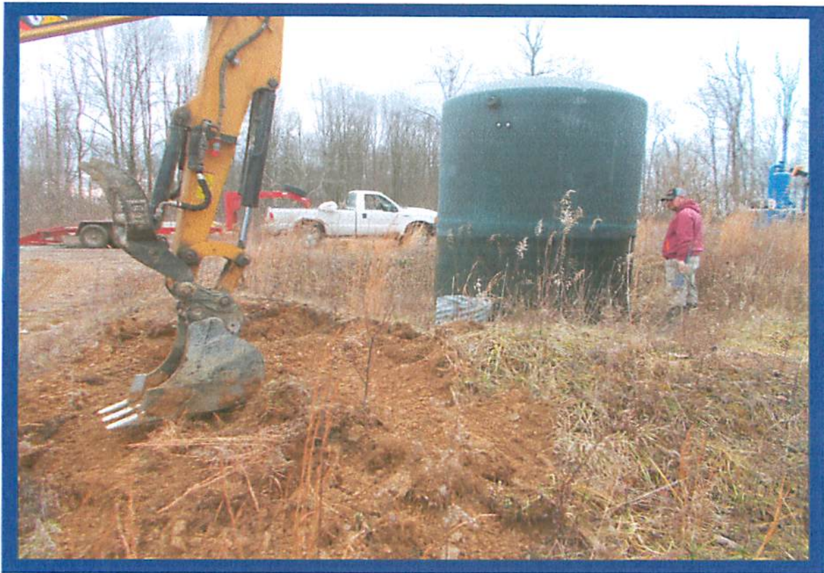
Photo 3: Discharge lines being uncovered to be removed.
