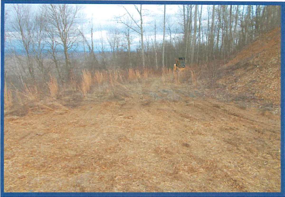
Photo 5: Tank location and dike area reclaimed.
