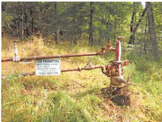
WV 656021 Well Pad Site
