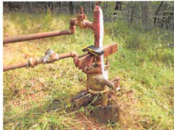
WV 656021 Well Pad Site
