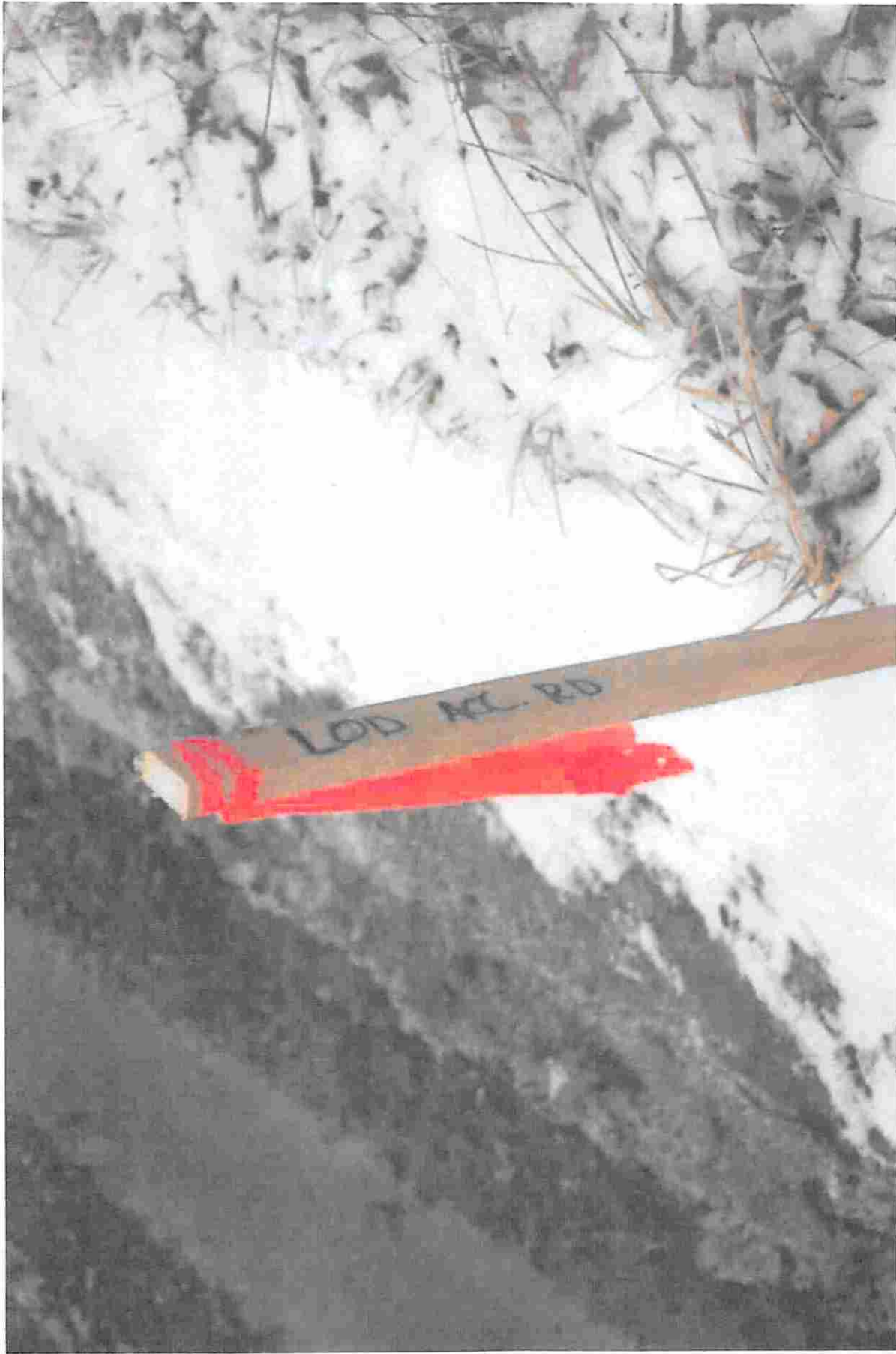
Detail of LOD marker on wrong side of property boundary
