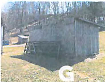
⬠ EXISTING STORAGE SHED
