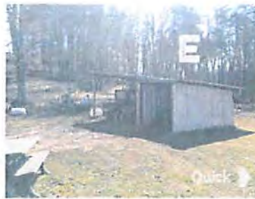
◇ EXISTING STORAGE SHED
