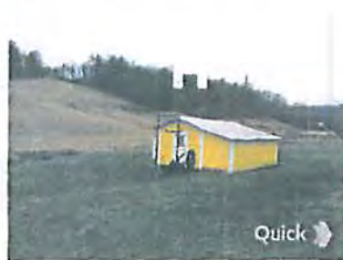
⬠ EXISTING STORAGE SHED
