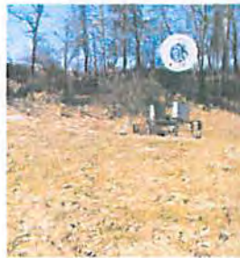
⬠ EXISTING PIPELINE METERS & LAUNCHERS
