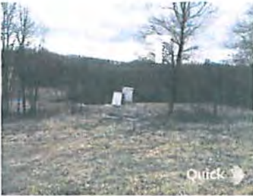
⬠ EXISTING PIPELINE METERS & PIG LAUNCHERS
