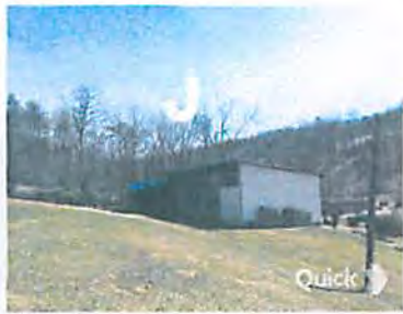
◇ EXISTING STORAGE SHED
