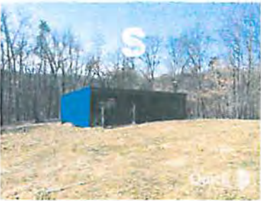
⬠ EXISTING STORAGE SHED
