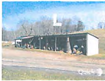
◇ EXISTING STORAGE SHED
