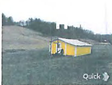
◊ EXISTING STORAGE SHED
