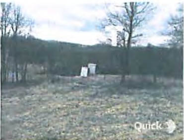
◊ EXISTING PIPELINE METERS & PIG LAUNCHERS
