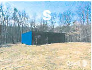
◊ EXISTING STORAGE SHED
