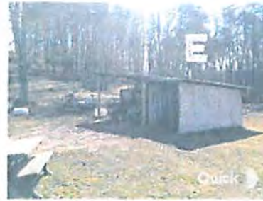
◇ EXISTING STORAGE SHED
