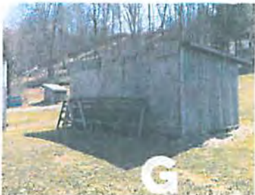
◊ EXISTING STORAGE SHED
