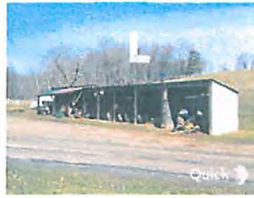
◇ EXISTING STORAGE SHED
