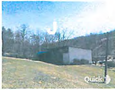
◇ EXISTING STORAGE SHED
