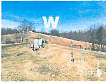
◇ EXISTING GAS WELL EQUIPMENT
