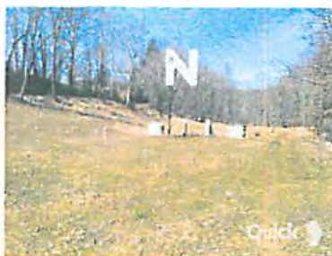
⬠ EXISTING GAS WELL EQUIPMENT
