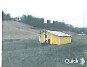
⬠ EXISTING STORAGE SHED
