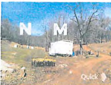
⬠ EXISTING GAS WELL EQUIPMENT ⬠ EXISTING TRUCK TRAILER
