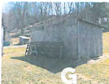
⬠ EXISTING STORAGE SHED
