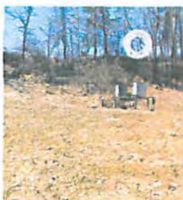
⬠ EXISTING PIPELINE METERS & LAUNCHERS
