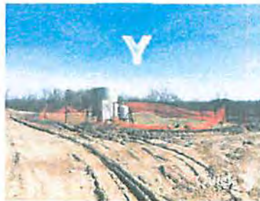
Y EXISTING GAS WELL PAD
