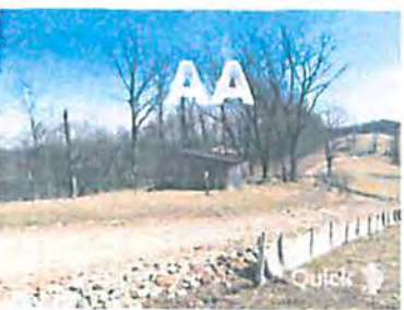
⬠ EXISTING STORAGE SHED
