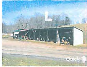
L EXISTING STORAGE SHED
