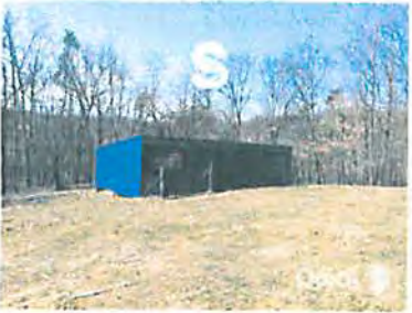
⬠ EXISTING STORAGE SHED
