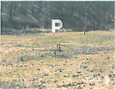
P EXISTING PIPELINE RISER
