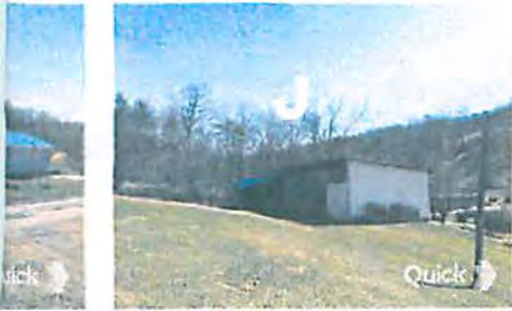
◇ EXISTING STORAGE SHED
