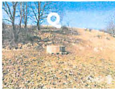
◇ EXISTING WATER TROUGH
