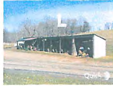
◇ EXISTING STORAGE SHED
