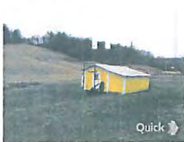
Ⓗ EXISTING STORAGE SHED
