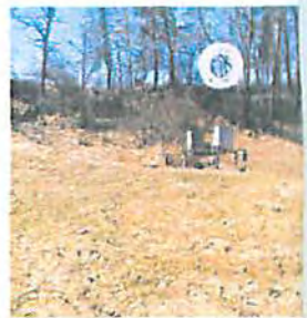
Ⓞ EXISTING PIPELINE METERS & PIG LAUNCHERS
