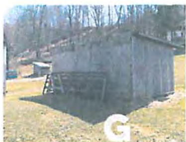
Ⓖ EXISTING STORAGE SHED
