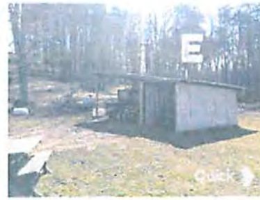
◇ EXISTING STORAGE SHED
