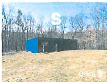
Ⓢ EXISTING STORAGE SHED
