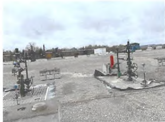
WEU4 Well Pad Site
