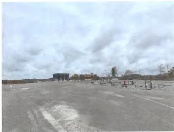
WEU4 Well Pad Site
