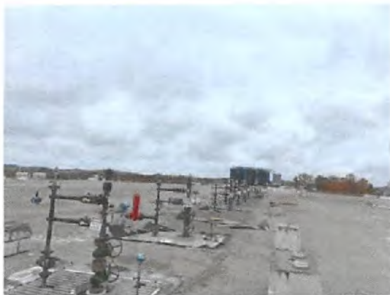
WEU4 Well Pad Site
