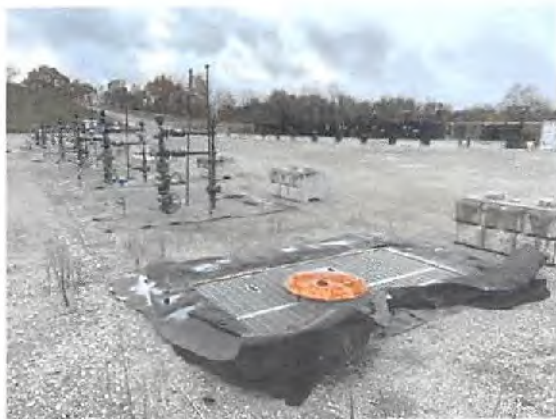
WEU4 Well Pad Site
