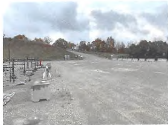
WEU4 Well Pad Site
