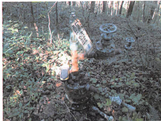
WV 452061 Well Pad Site
