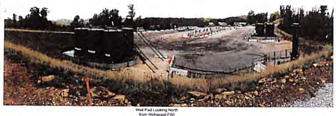
Well Pad Looking North from Richwood P.01
