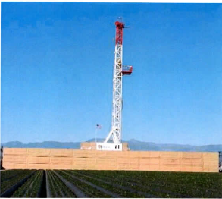
Figure 1. A sound blanket surrounding the drill rig would not work very well for obvious reasons. Source: https://www.drillingnoisecontrol.com/drilling-rig-sound-control-systems/temporary-perimeter-sound-walls/ .
