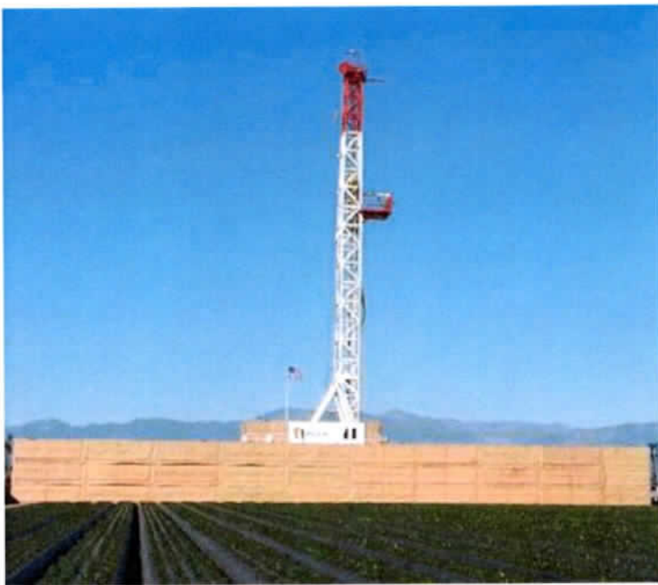
Figure 1. A sound blanket surrounding the drill rig would not work very well for obvious reasons. Source: https://www.drillingnoisecontrol.com/drilling-rig-sound-control-systems/temporary-perimeter-sound-walls/ .
