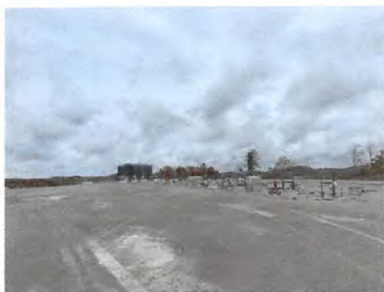
WEU4 Well Pad Site
