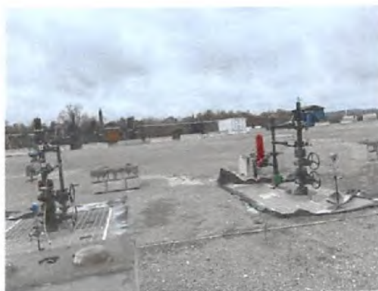
WEU4 Well Pad Site
