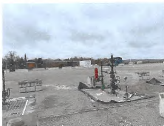
WEU4 Well Pad Site
