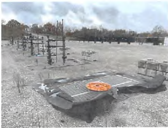
WEU4 Well Pad Site
