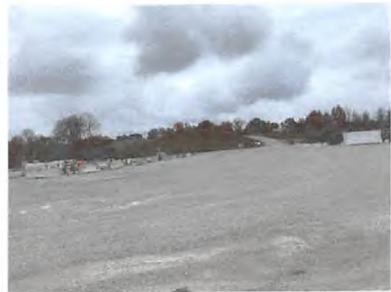
WEU4 Well Pad Site
